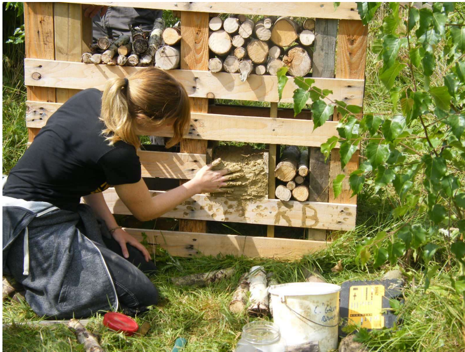
Fig 3. Bee and bug hotel under construction; two pallets were screwed together and materials stuffed into the gaps including deadwood, bamboo canes, hay and clay.
